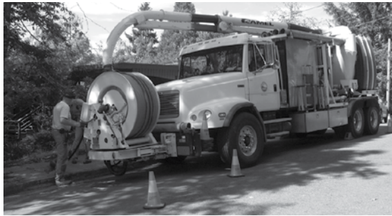
City crews clean storm drainage lines to keep them flowing freely
