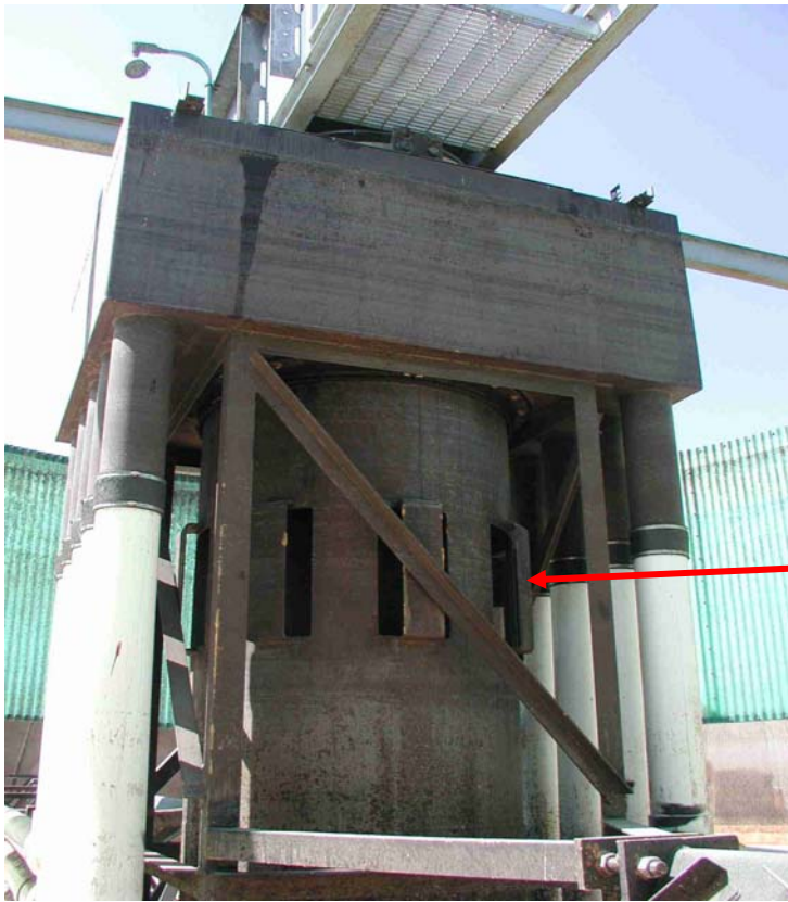
FIGURE 1 Existing Secondary Clarifier Center Column MWMC Facility Plan, Eugene-Springfield
